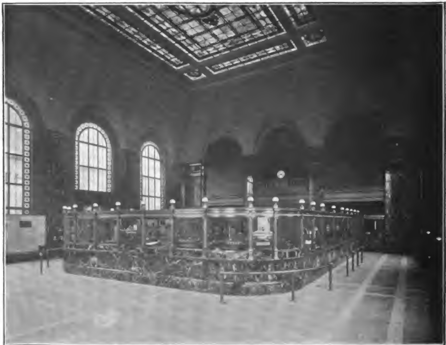
New Building of the Springfield (Mass.) Institution for Savings.
